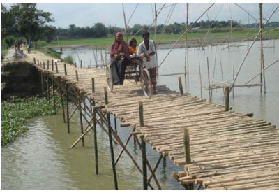
Bamboo Bridge in Shahadebpur, Kalihati improvement Training in Narandia
